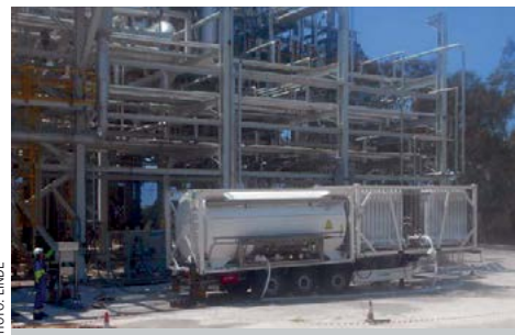
Fig. 2: Mobile oxygen supply chain based on liquid oxygen.
