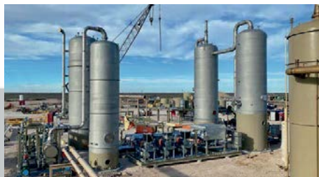
Below: Large Valkyrie™ plant under construction.
