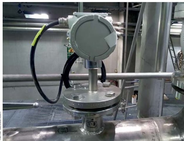
Fig. 2: LiquiSonic® inline immersion sensor.
