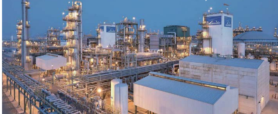
The Sadara Chemical Company complex, Al Jubail, Saudi Arabia.
