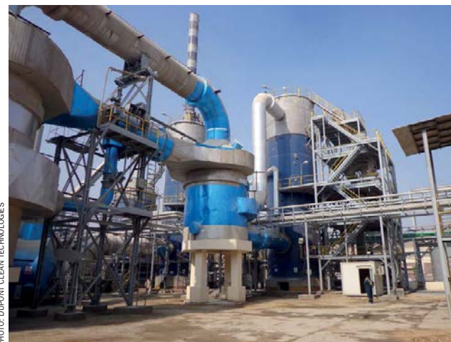
AZFC's Unit 6 after the revamp project.
