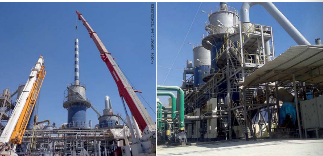
Left: The new tower as it is lifted into place at Unit 6. Right: Since start-up, Unit 6 has operated to performance guarantees, producing up to 640 t/d of acid.
