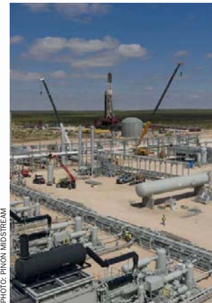
Piñon Midstream's Dark Horse facility under construction.
