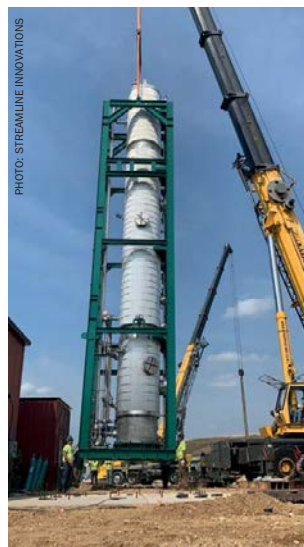
Packed tower installation.
