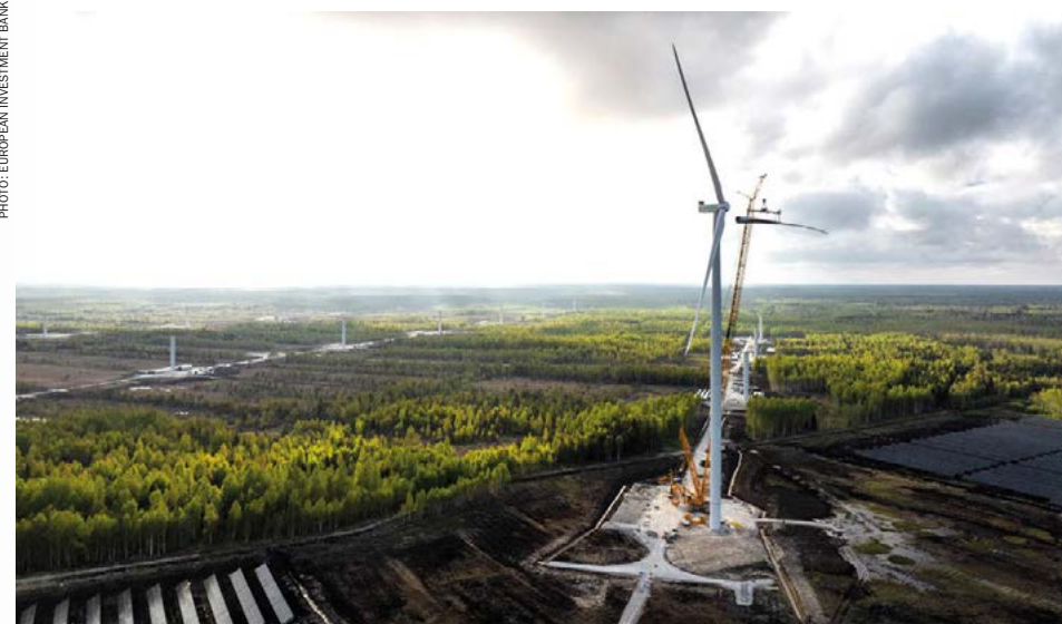
Installing new onshore wind turbines in Denmark.
