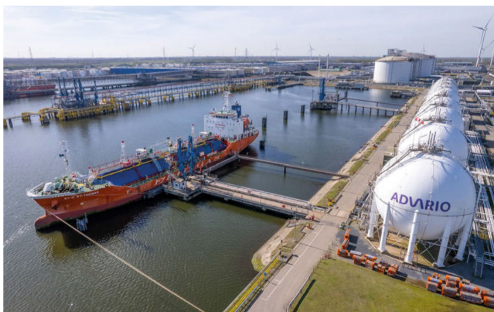
Fluxys is building a new ammonia import terminal at Advario's Gas Terminal at Antwerp, part of Europe's projected needs for higher ammonia imports in future.
