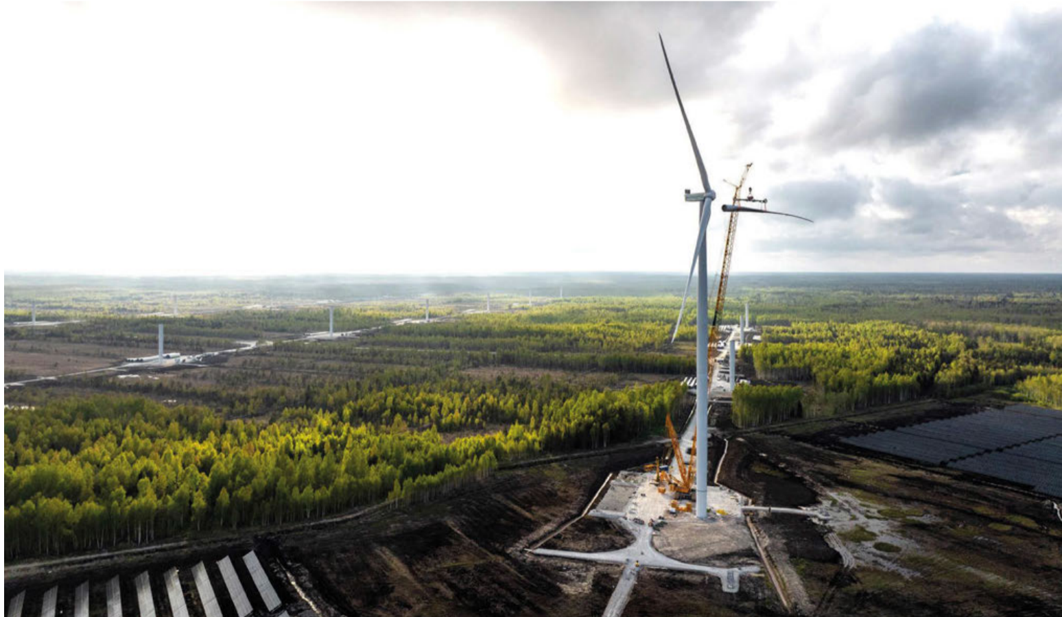
Installing new onshore wind turbines in Denmark.
