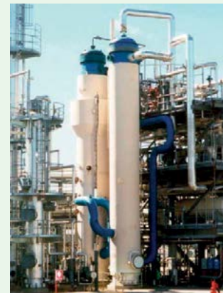
Fig. 5: Gas heated reformer (GHR) and secondary reformer at Coogee, Australia.
