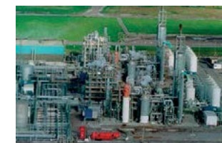
Fig. 1: The two LCA plants at Sevenside (shutdown 2008).
