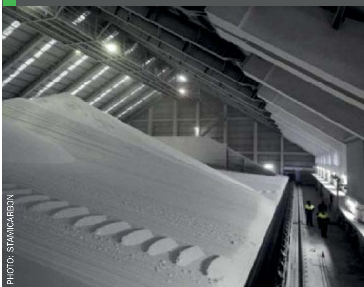
Fig. 3: Bulk storage of urea
