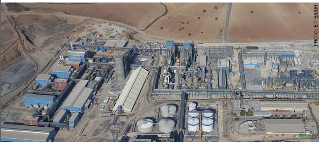
Eti Bakir's new Mazidagi Phosphate plant provides around 0.7 million tonnes of additional DAP/NP capacity.
