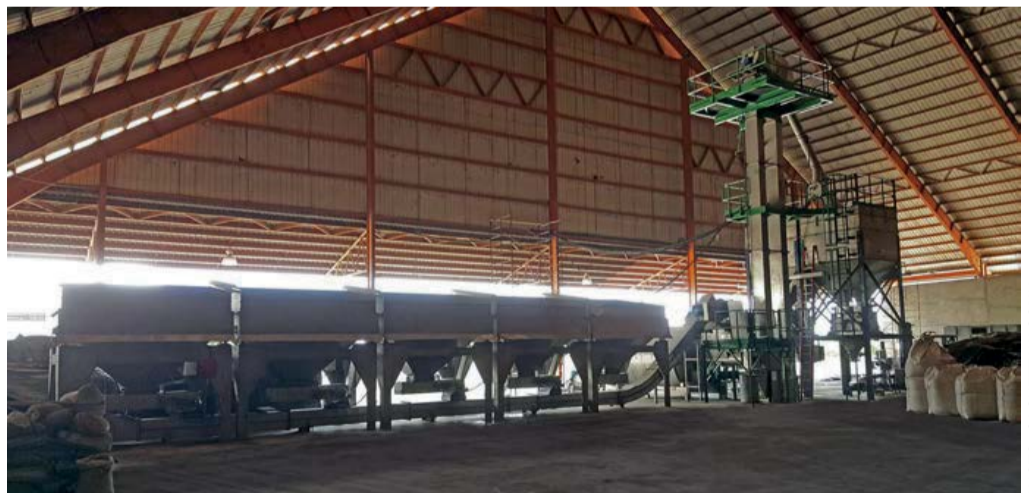
Sackett-Waconia Precision Horizontal Blending system for Mayafert, Guatemala.
