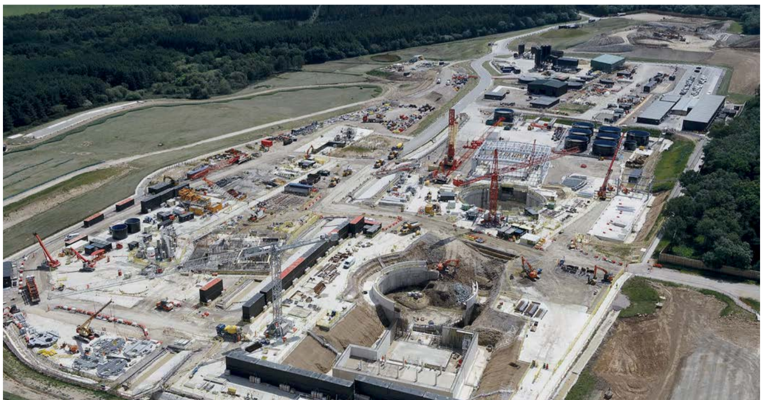
The under-construction Woodsmith mine near Whitby, North Yorkshire, UK.
