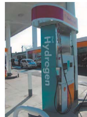
Hydrogen filling station, California.
