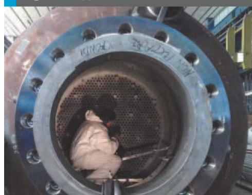
Fig 6: Stripper construction
