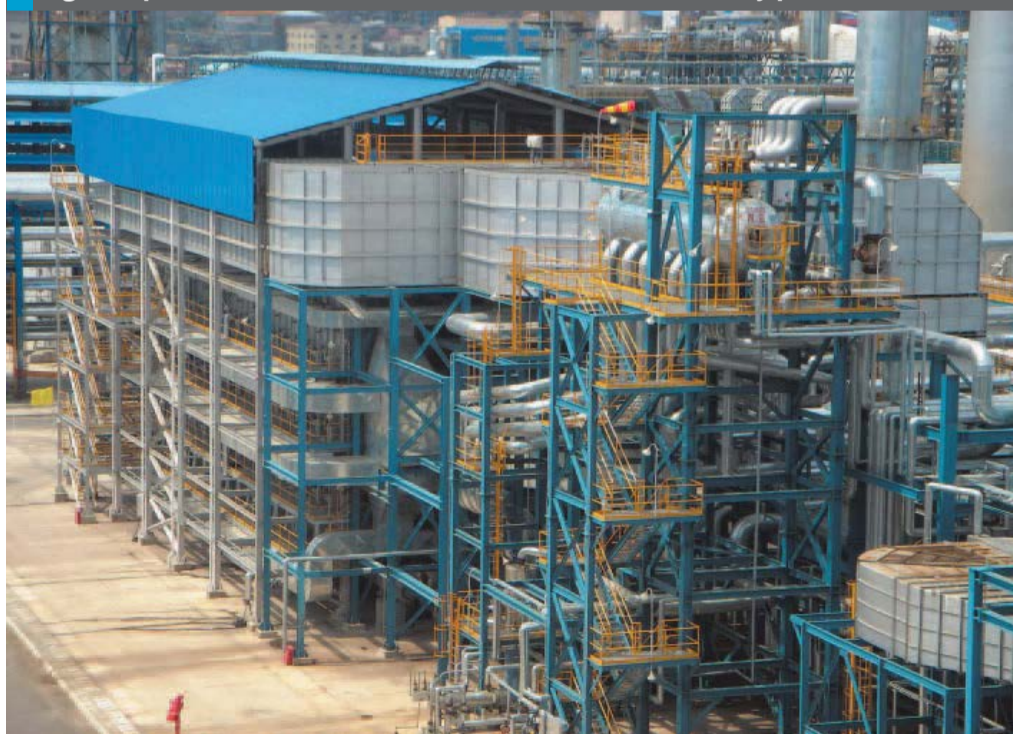
Fig 1: Topsoe side-fired steam reformer – waste heat recovery placed at side
