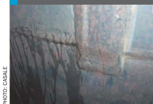
Fig 3: Impingement damage on titanium
