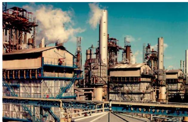
Fig. 5: Three 1,000 t/d Kellogg plants built at Billingham.
