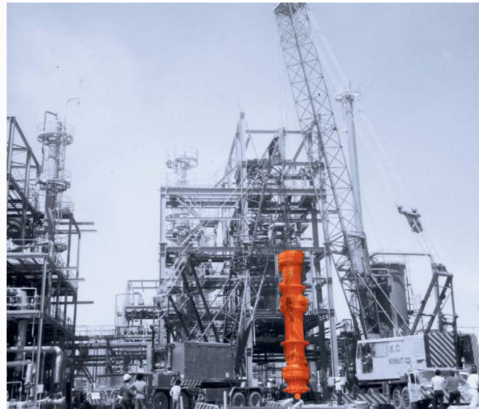
Late seventies, Kuwait Melamine plant under construction
