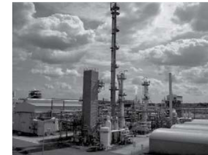
13,200 Nm 3 /hr Hydrogen Plant
