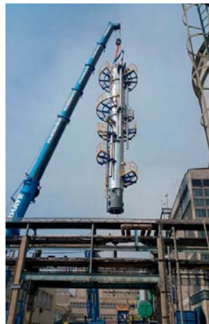
Fig 1: Installation of new saturation tower.
