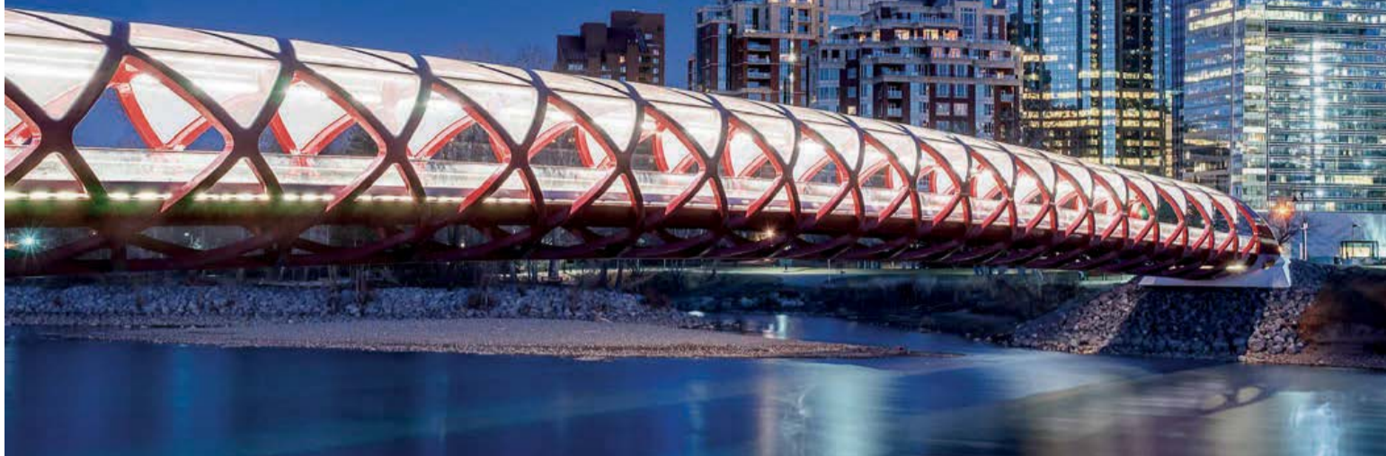
Peace Bridge, Calgary, is a pedestrian bridge, designed by Spanish architect Santiago Calatrava.
