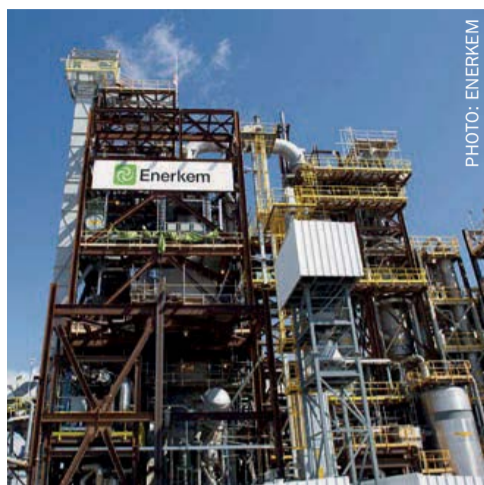
Enerkem's waste to methanol facility, Edmonton, Alberta.
