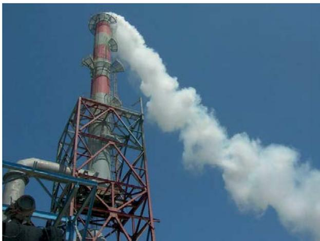
Start-up plume from a sulphuric acid plant.
