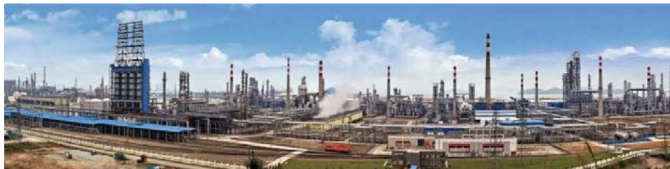
Fig. 5: CNOOC Huizhou Refinery in Guangdong, China.
