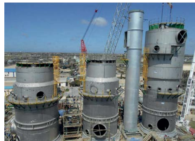
Fig. 7: NORAM SX™ alloy acid towers.
