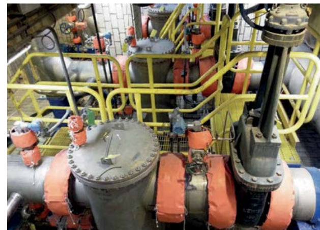
Fig. 6: NORAM SX™ Chip Guard CG™ in-line strainer.
