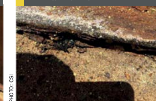
Fig. 11: Typical tank floor surface with bottom-up corrosion near perimeter
